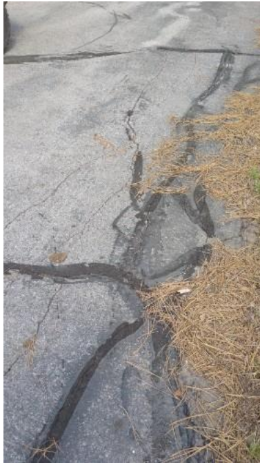
Smaller cracks that were properly sealed
