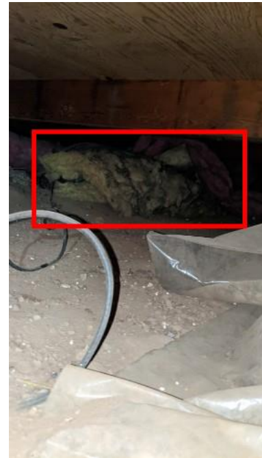
Displaced insulation
