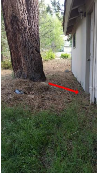
Slopes towards garage access door and East side of home.
