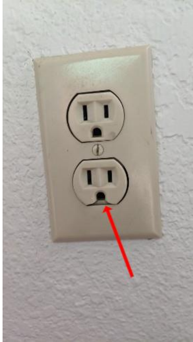
Damaged outlet
