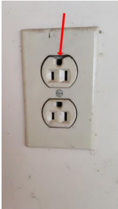
Damaged outlet
