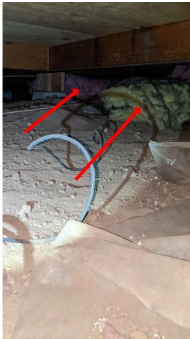
Displaced insulation
