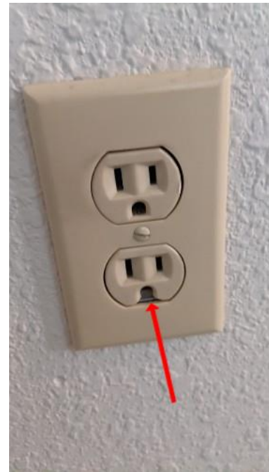
Damaged outlet
