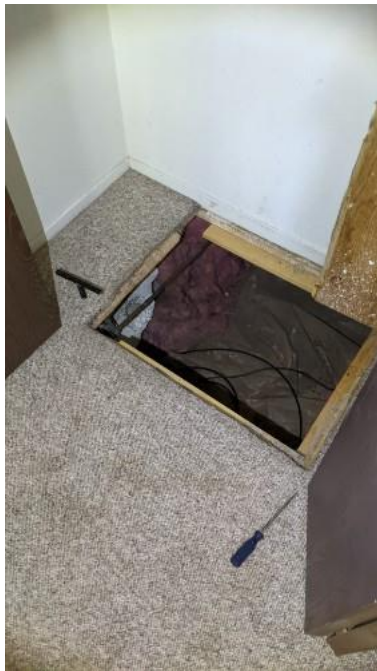
2nd crawlspace access in Southeast corner bedroom
