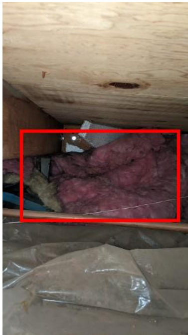
Displaced insulation
