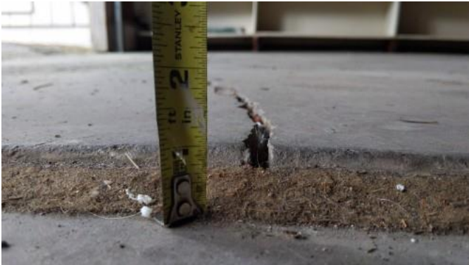
Middle divider of the two car garage is raised nearly an inch
