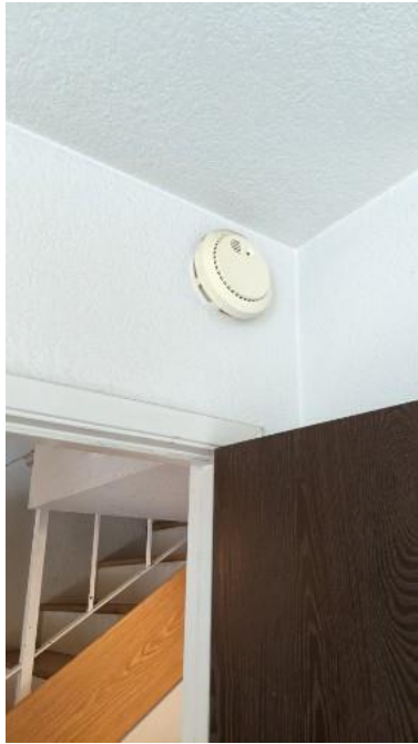
Primary BR - no response when tested
