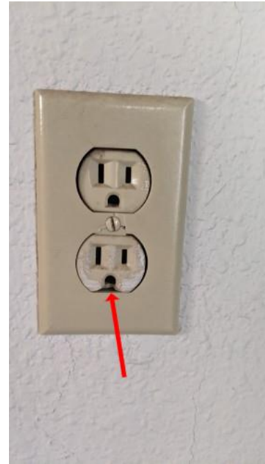
Damaged outlet
