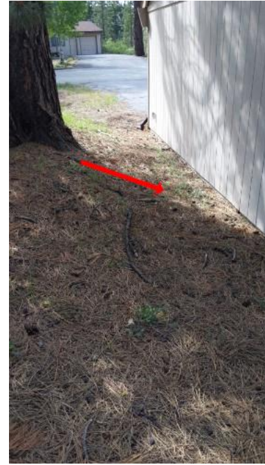
Slopes towards South side of the home/garage.
