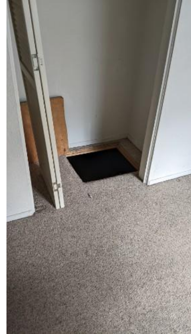
Crawlspace access in primary bedroom closet
