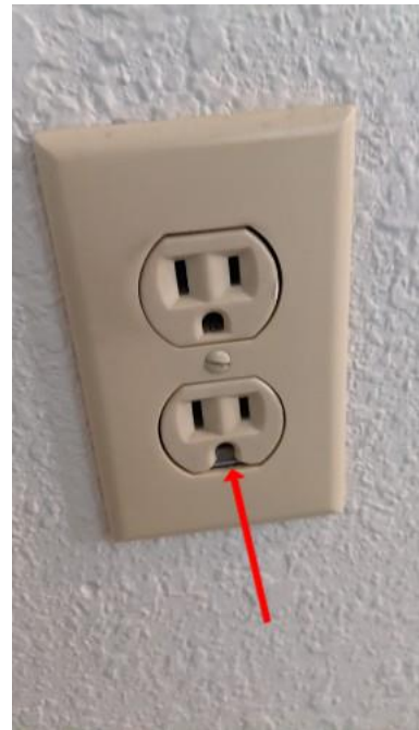
Damaged outlet
