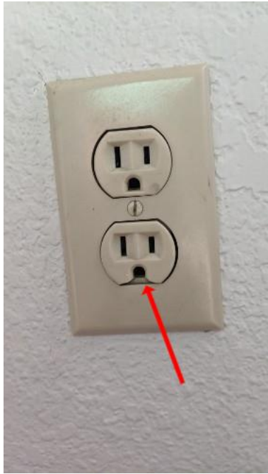
Damaged outlet
