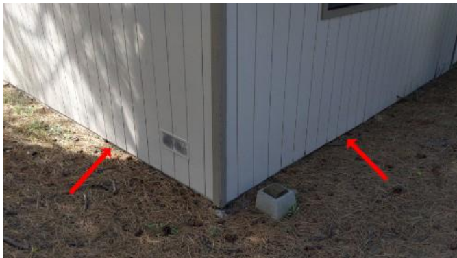
View of both East and South side exterior
