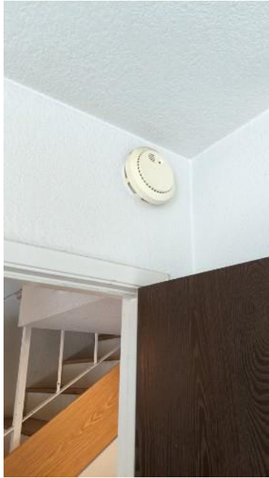
Primary BR - no response when tested
