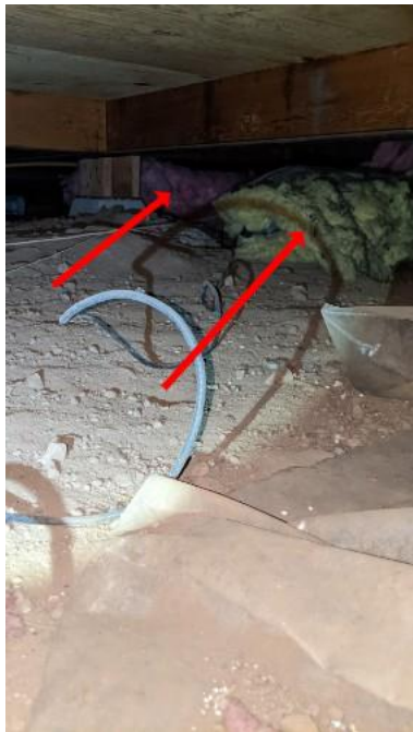
Displaced insulation
