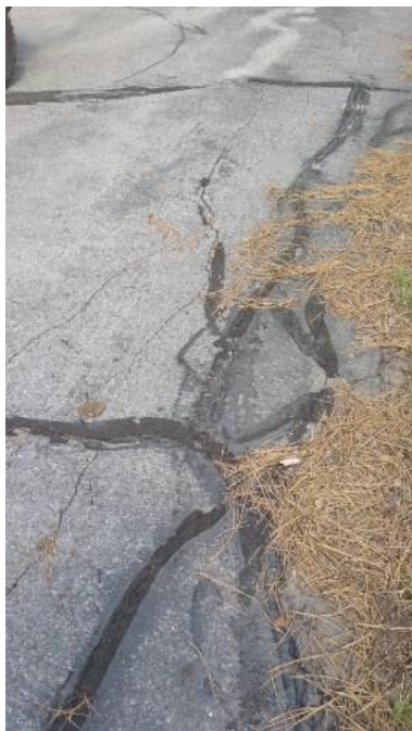
Smaller cracks that were properly sealed
