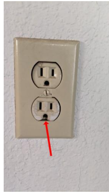
Damaged outlet
