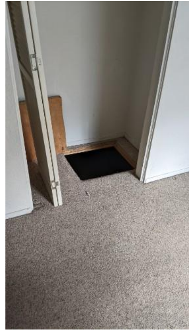
Crawlspace access in primary bedroom closet
