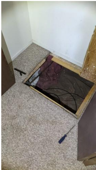
2nd crawlspace access in Southeast corner bedroom
