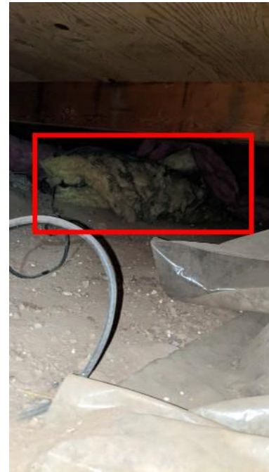
Displaced insulation
