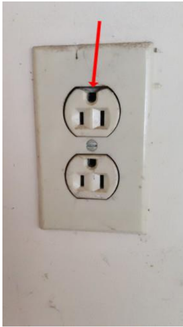
Damaged outlet
